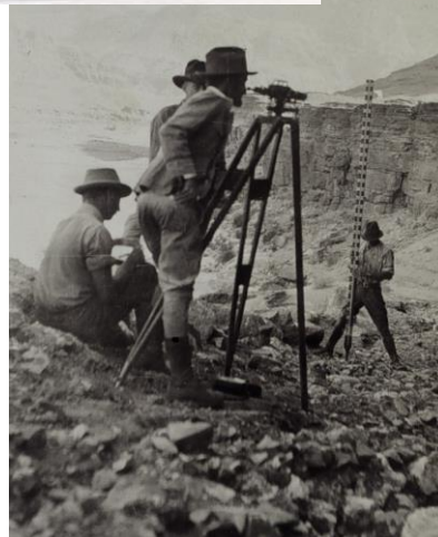
The first geodetic leveling - the beginning of the vertical control network - was along the Hudson River in 1856
